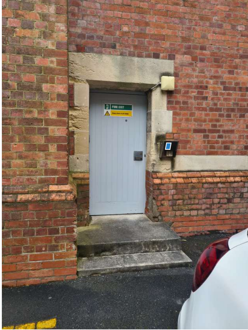
QR code by swipe access ACM Panel
