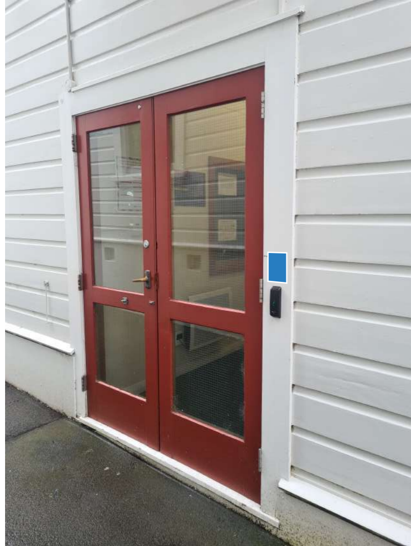
QR code by swipe access ACM Panel
