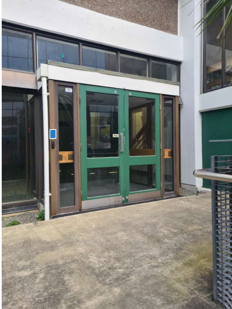
QR code by swipe access ACM Panel
