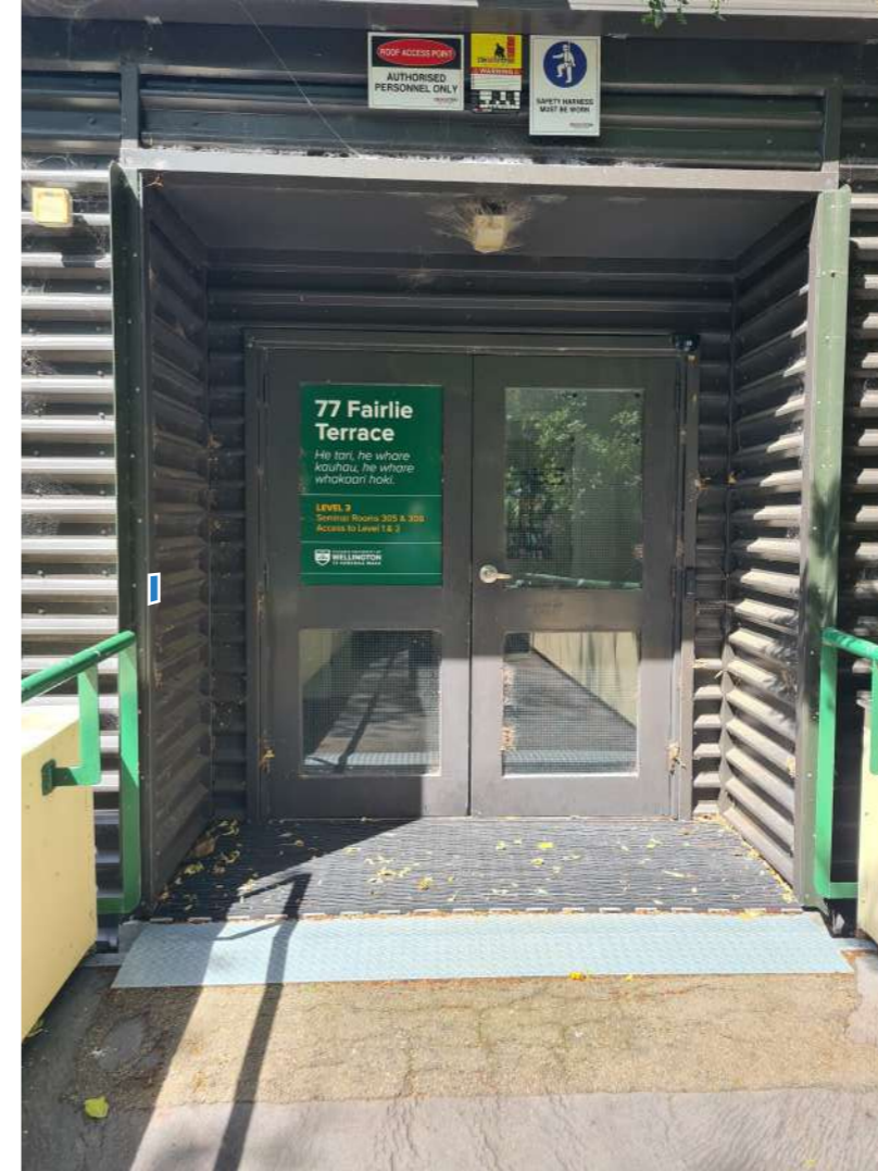
QR code on left side of door ACM Panel
