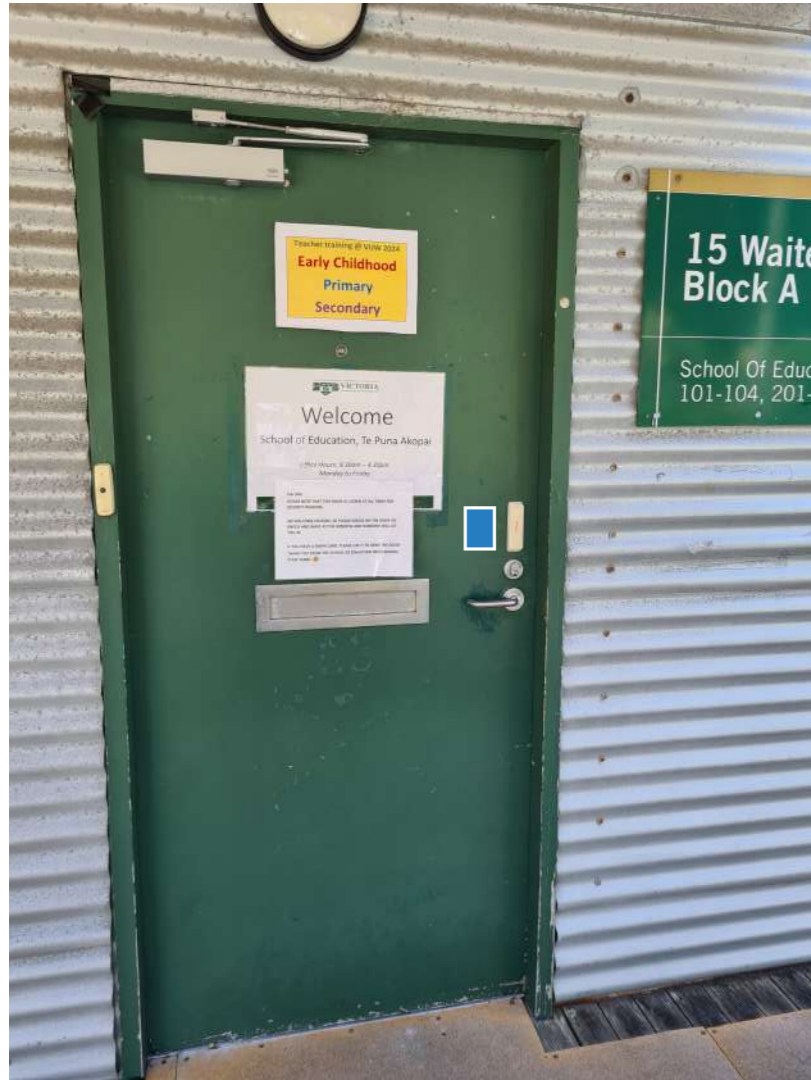
QR code by swipe access ACM Panel
