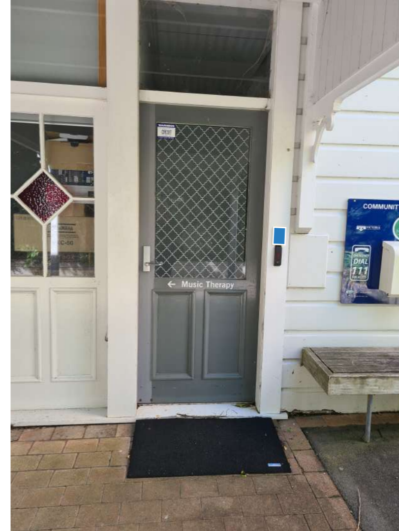
QR code by swipe access ACM Panel
