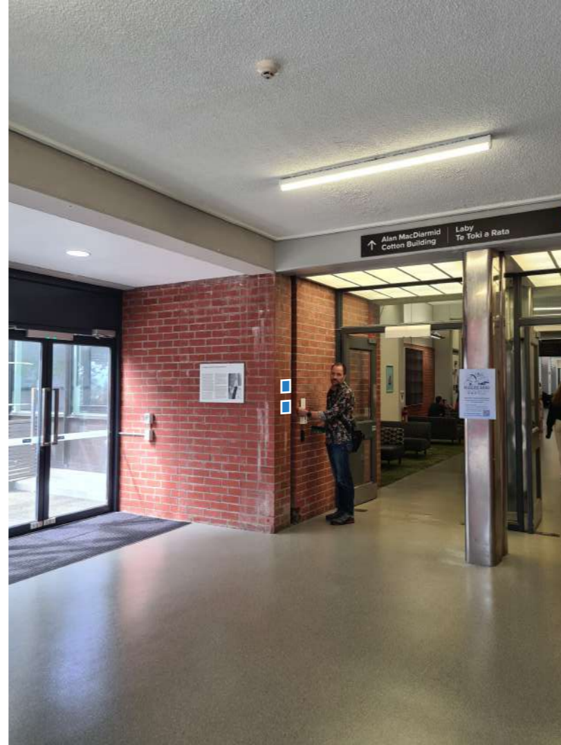
QR code by fire wall x2 ACM Panel
