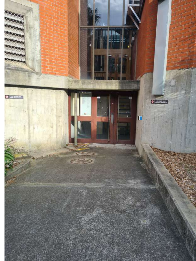
QR code by swipe access ACM Panel
