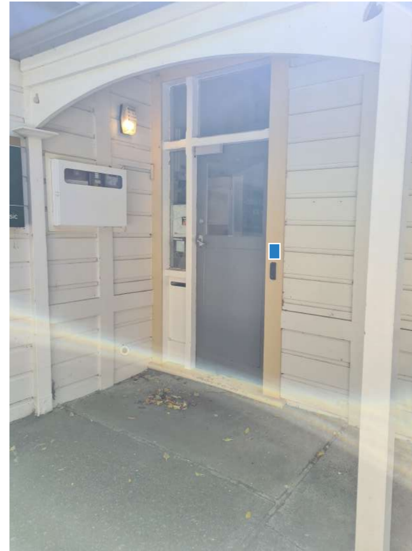
QR code by swipe access ACM Panel
