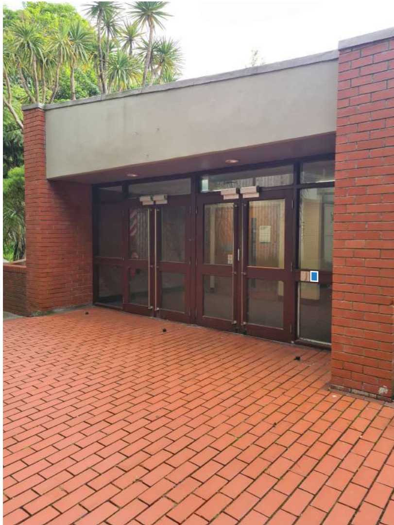
QR code by swipe access ACM Panel
