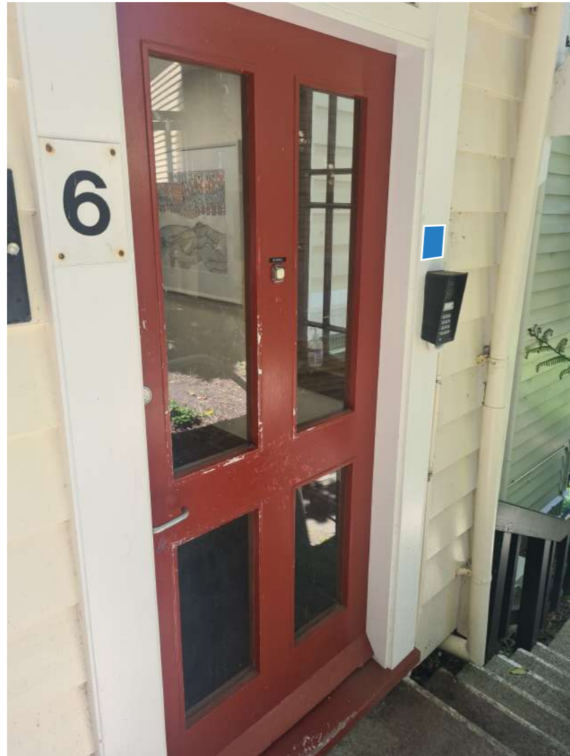
QR code by code access ACM Panel
