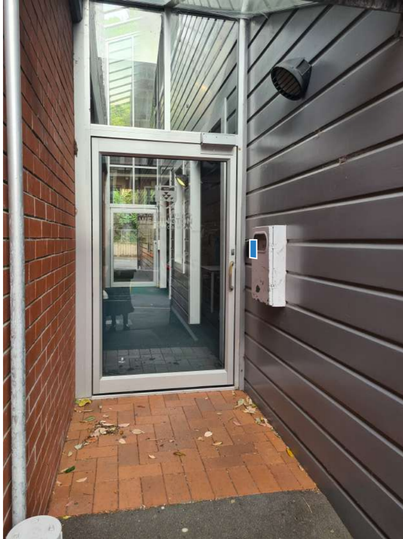
QR code by swipe access ACM Panel
