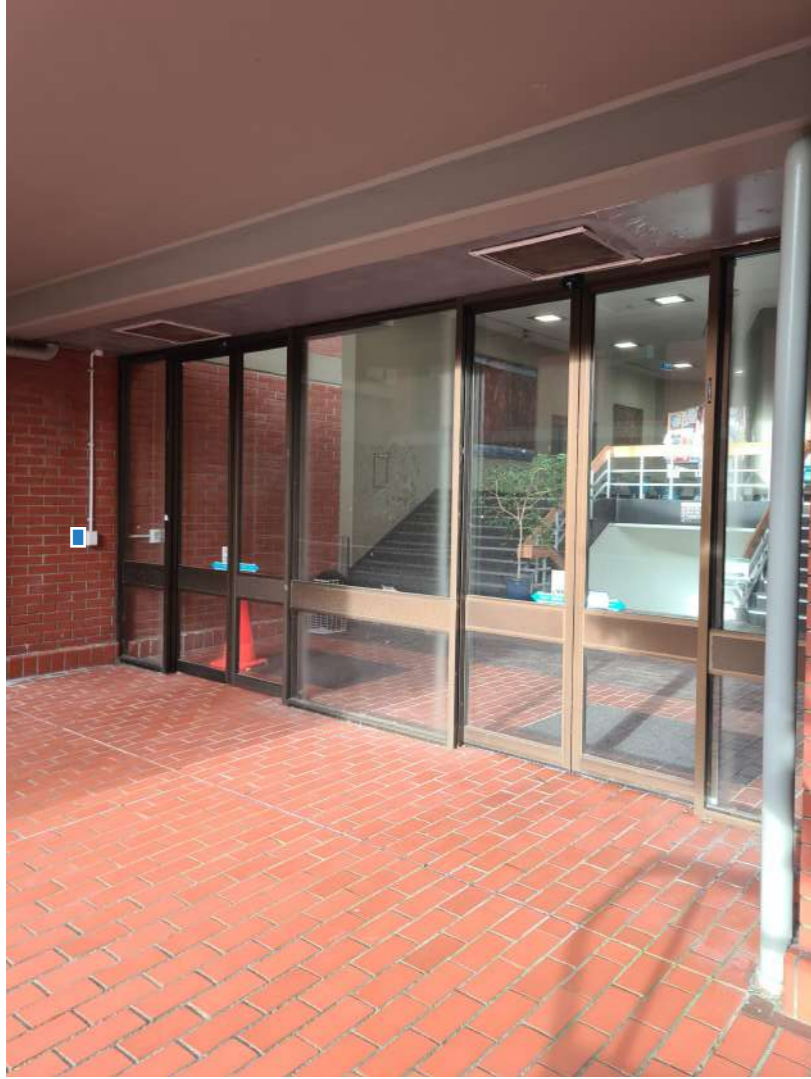
QR code by swipe access ACM Panel
