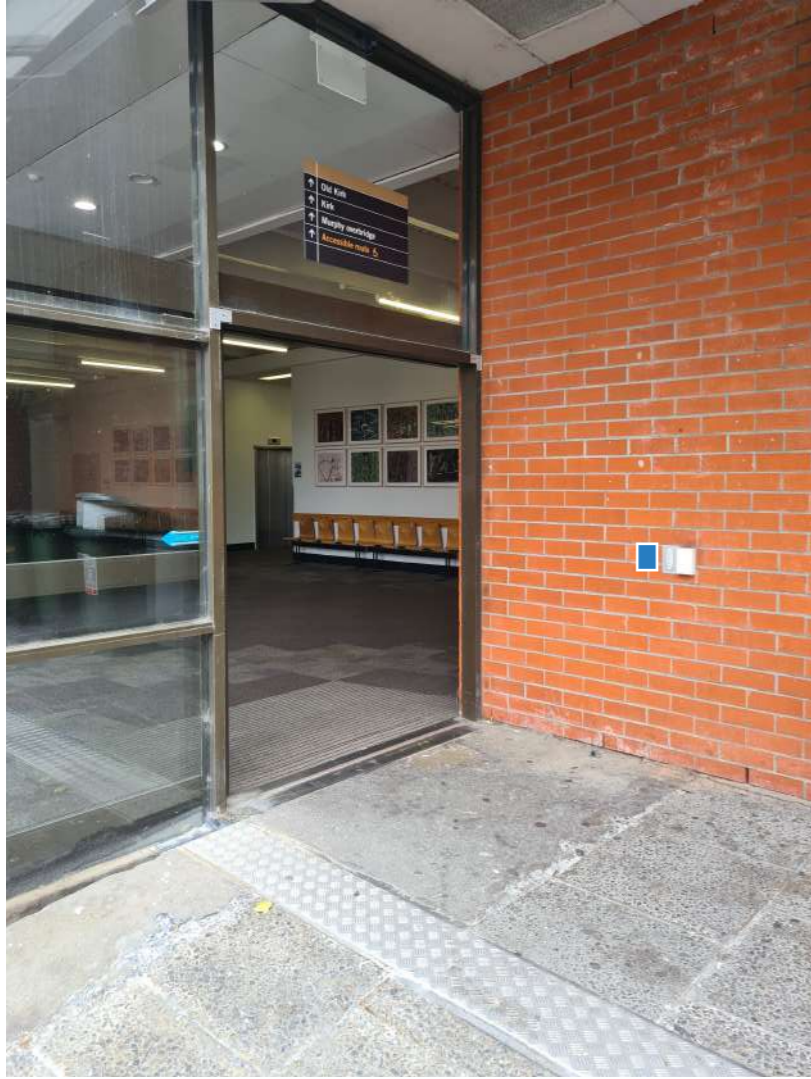
QR code by swipe access ACM Panel
