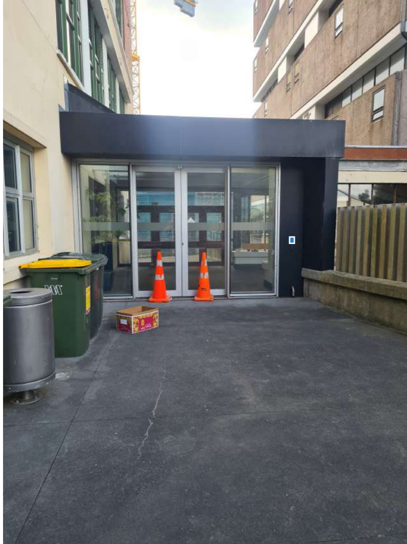
QR code by swipe access ACM Panel
