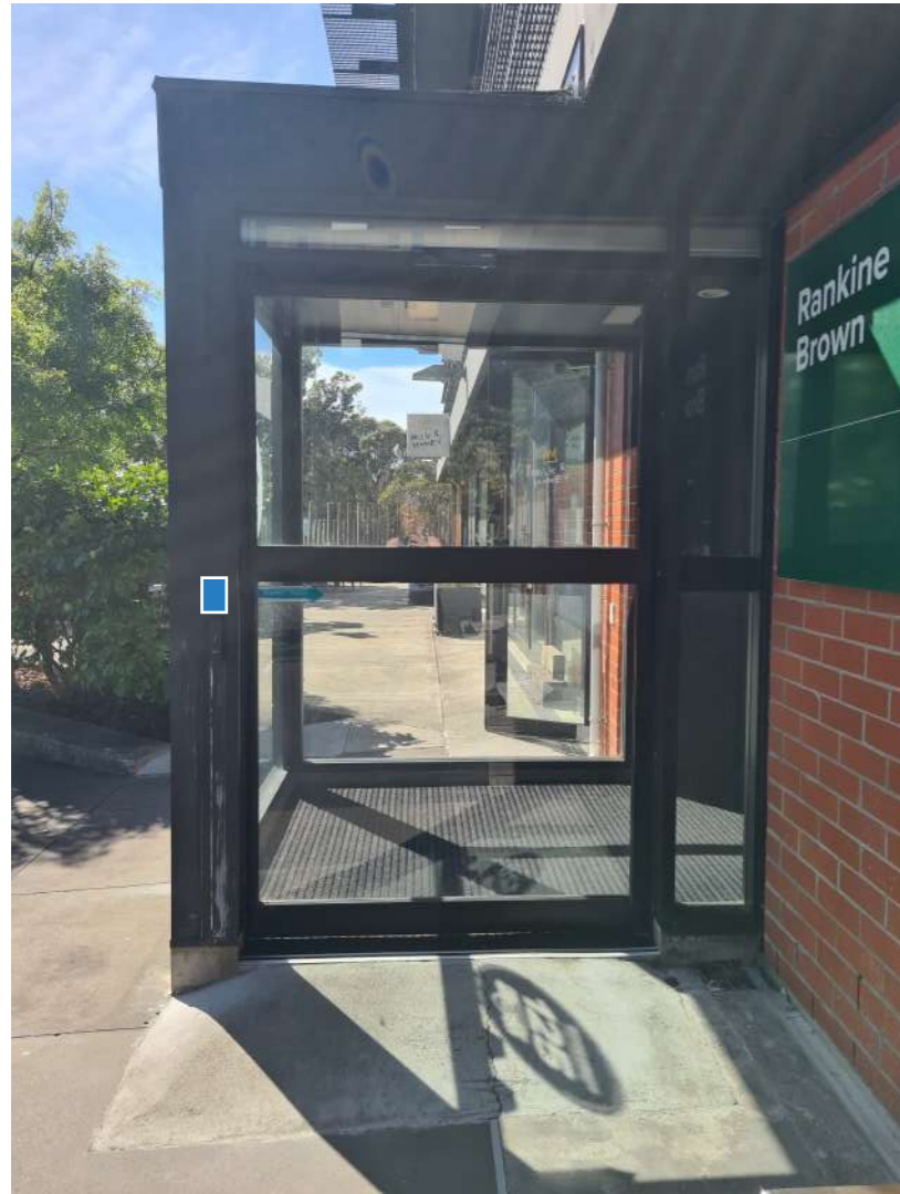
QR code by swipe access ACM Panel
