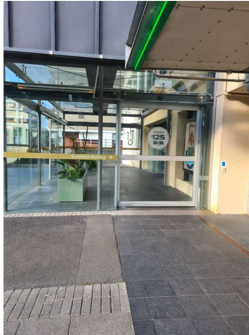
QR code by swipe access ACM Panel
