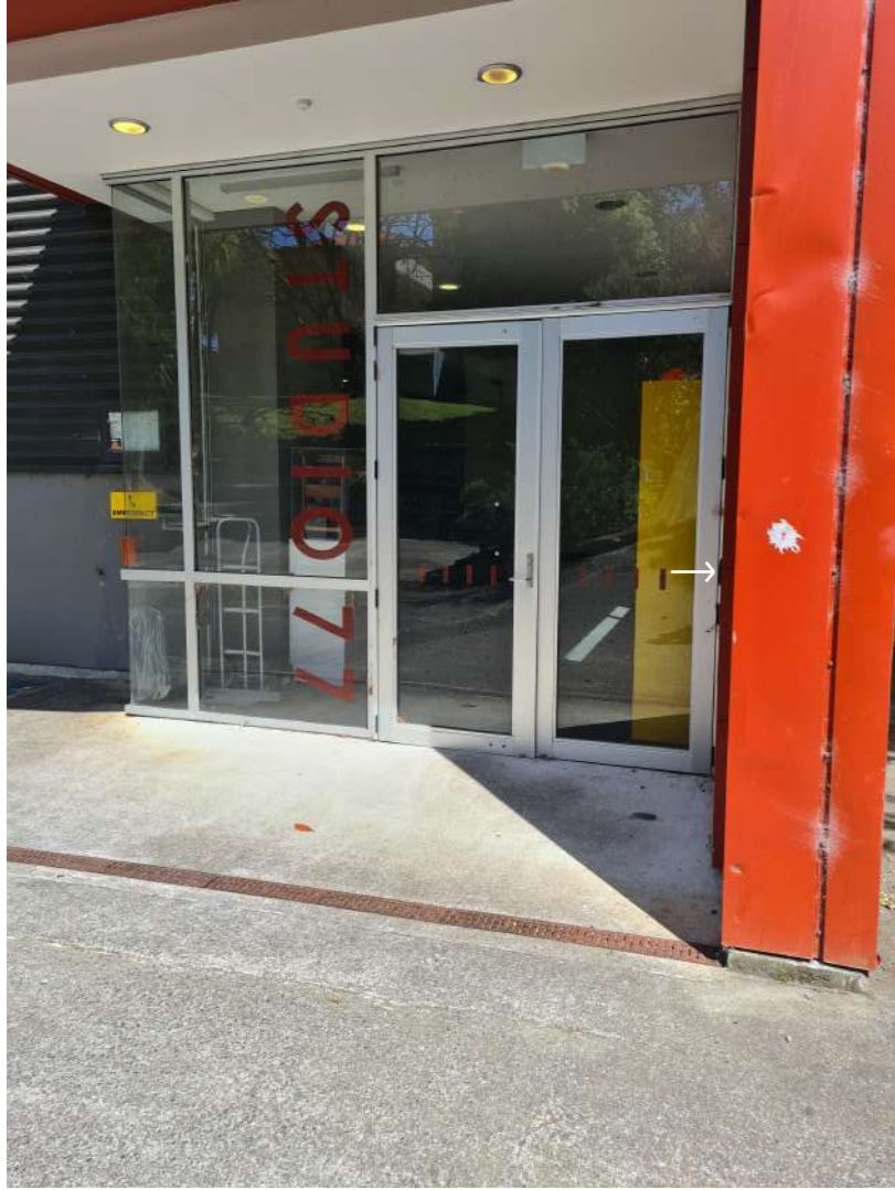
QR code by swipe access ACM Panel
