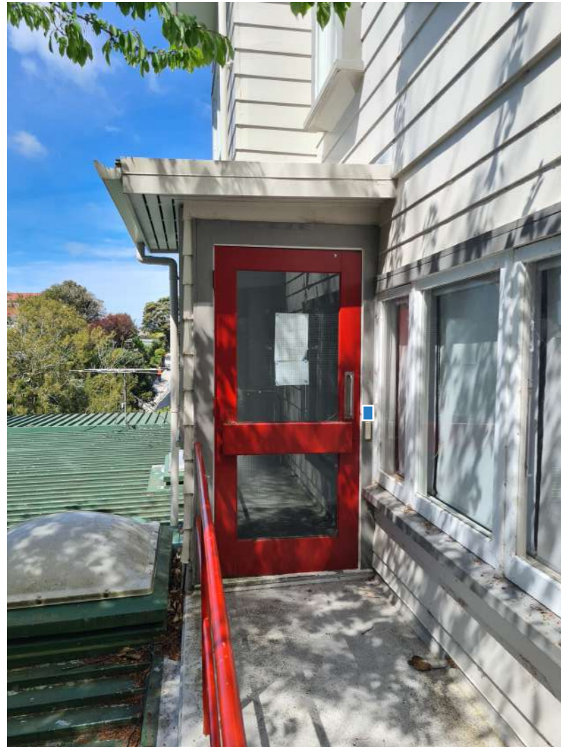
QR code by swipe access ACM Panel
