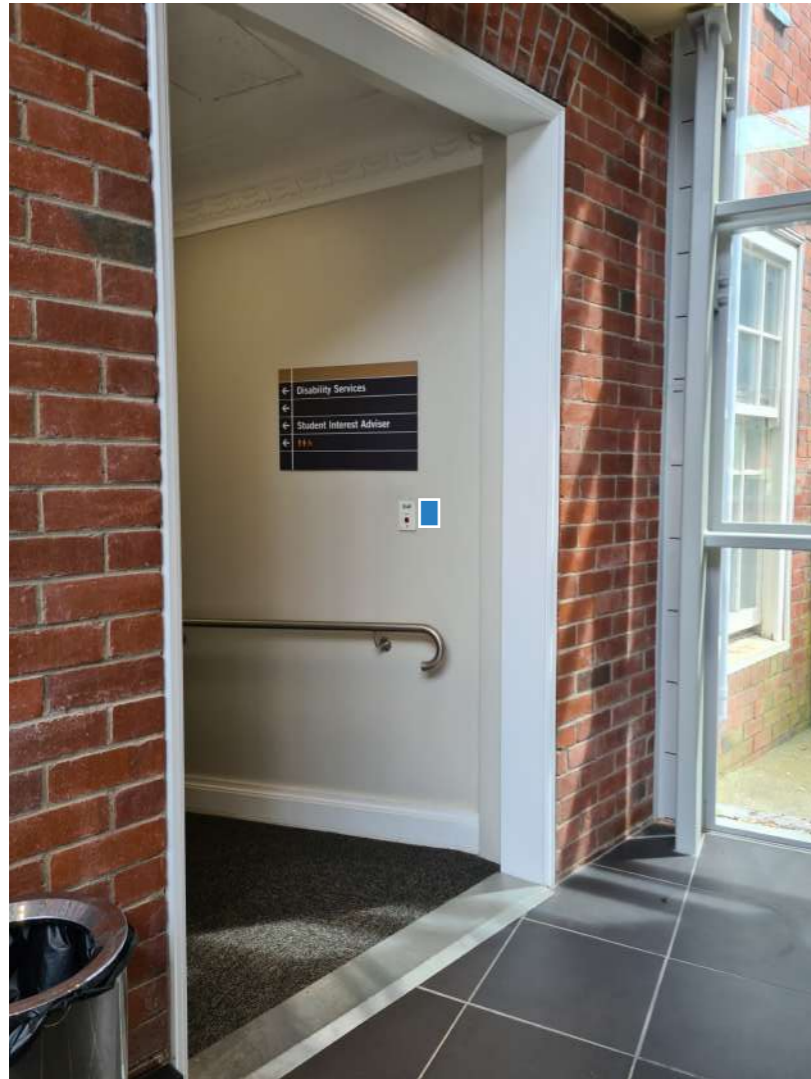
QR code by light switch ACM Panel
