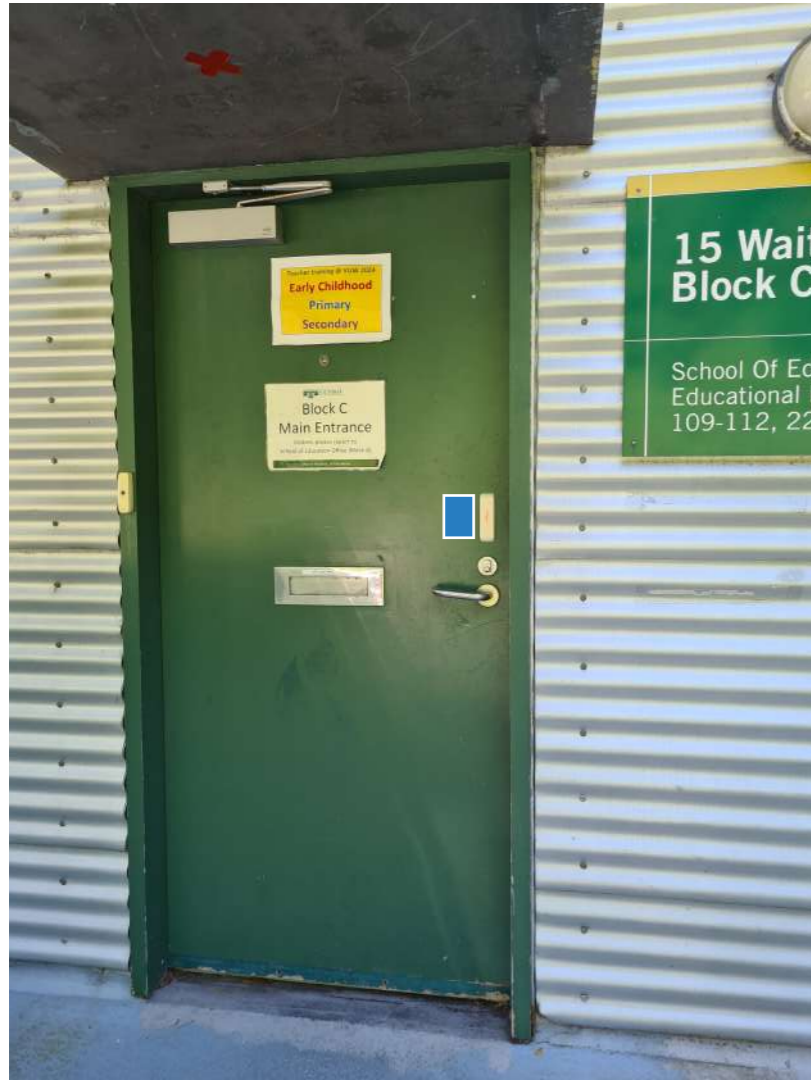
QR code by swipe access ACM Panel
