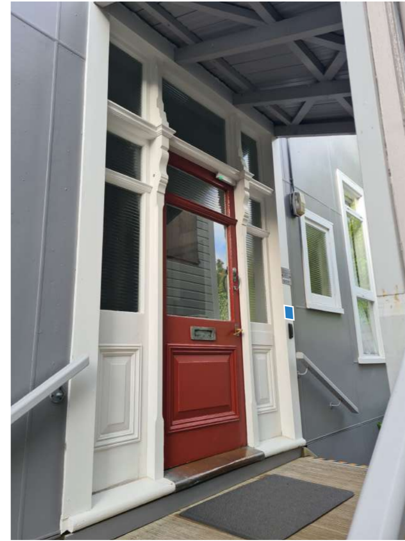
QR code by swipe access ACM Panel
