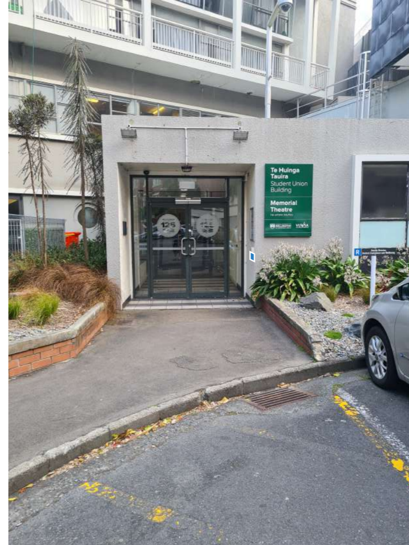
QR code by swipe access ACM Panel
