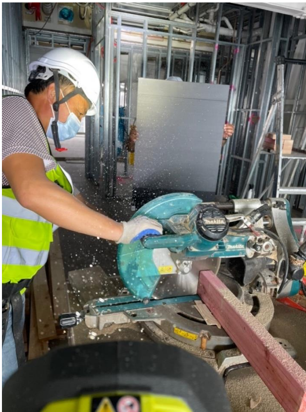
Figure 22: Case Study C - Construction Site, circular saw, breathing zone observation.
