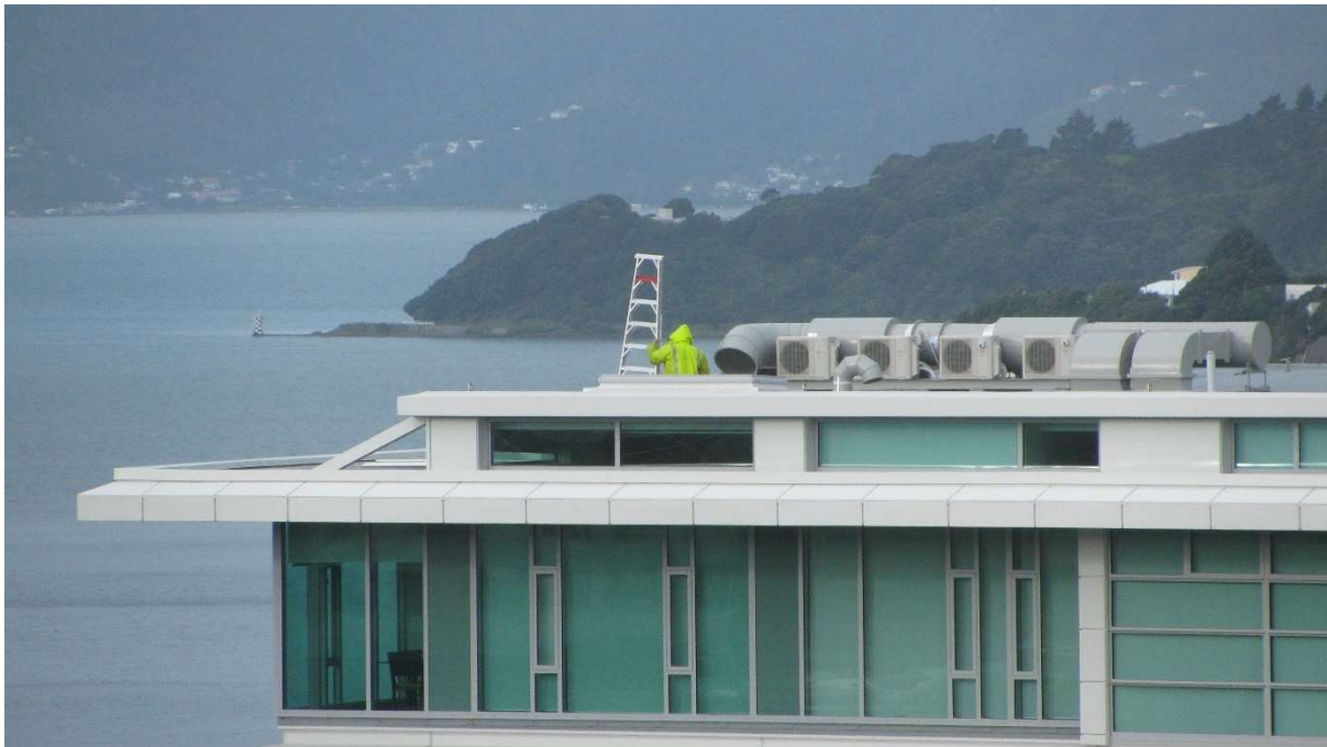
Figure 11: Worker bringing a ladder to access service areas at Chews Lane Apartments
