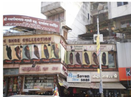
Fig. 8 Adjacent building with different heights, Pune.
