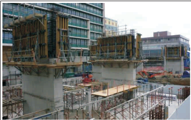
Fig. 1 General view of the site and the cantilevered reinforced concrete
