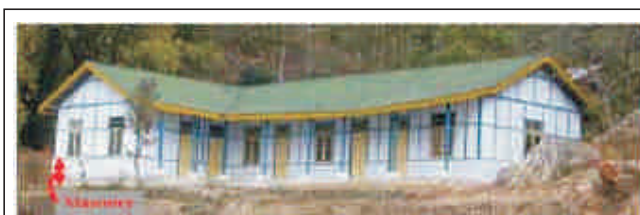
Fig. 4. Traditionally constructed typical Ikra structure in Sikkim (school building at Nandok, East Sikkim).
