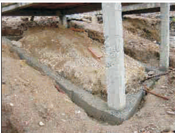
Fig. 9. Provision of grade beams on slope
